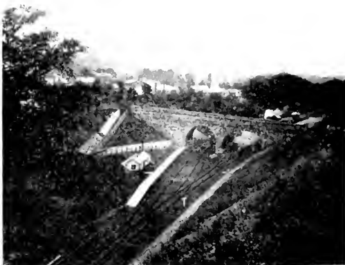
Holywell Town Station.
